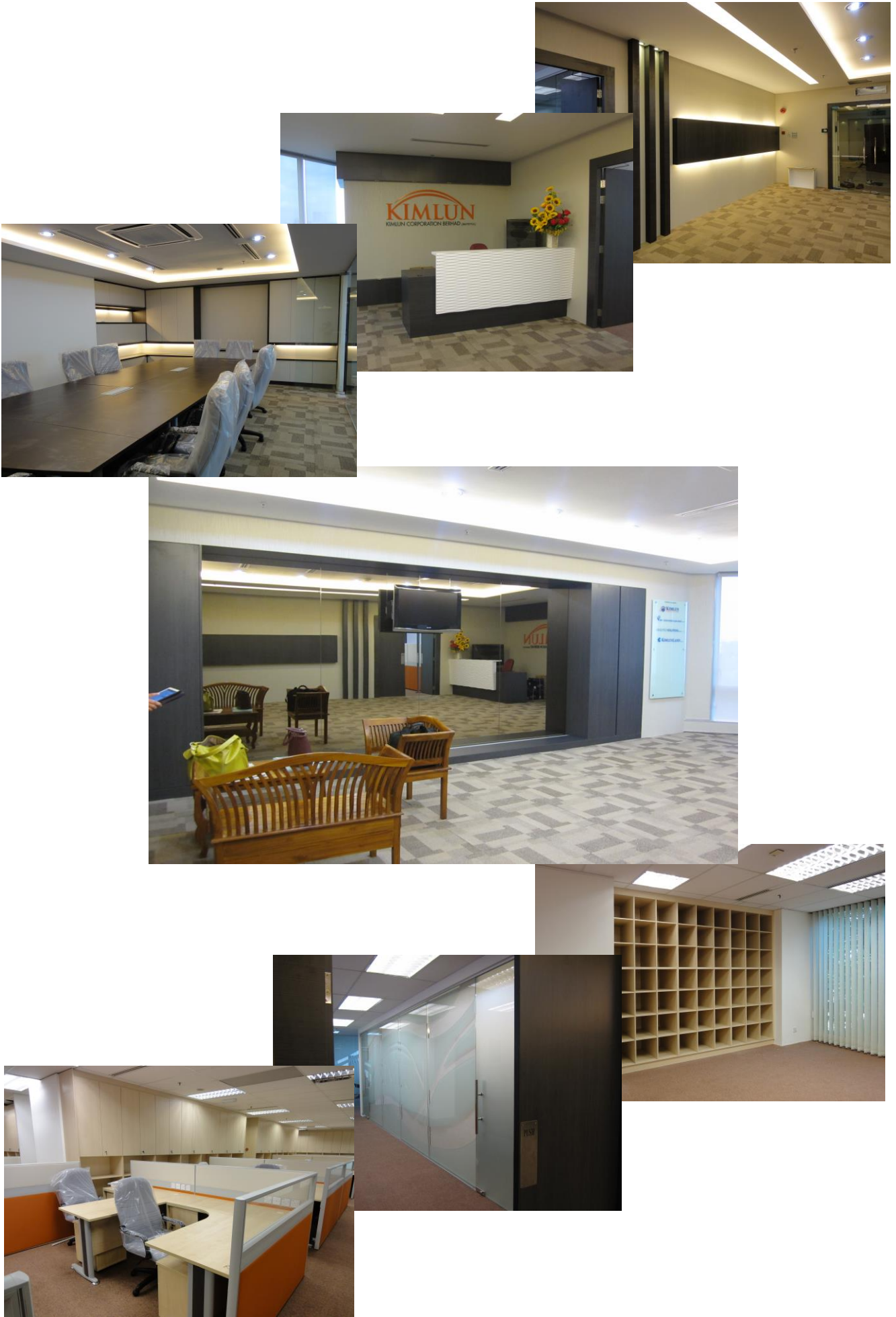
OFFICE RENOVATION WORK
